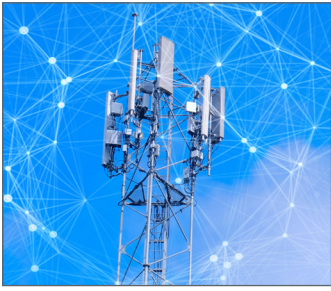
4G/5G Wireless Infrastructure
